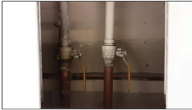
5.0 Item 1(Picture) Main water shut off
